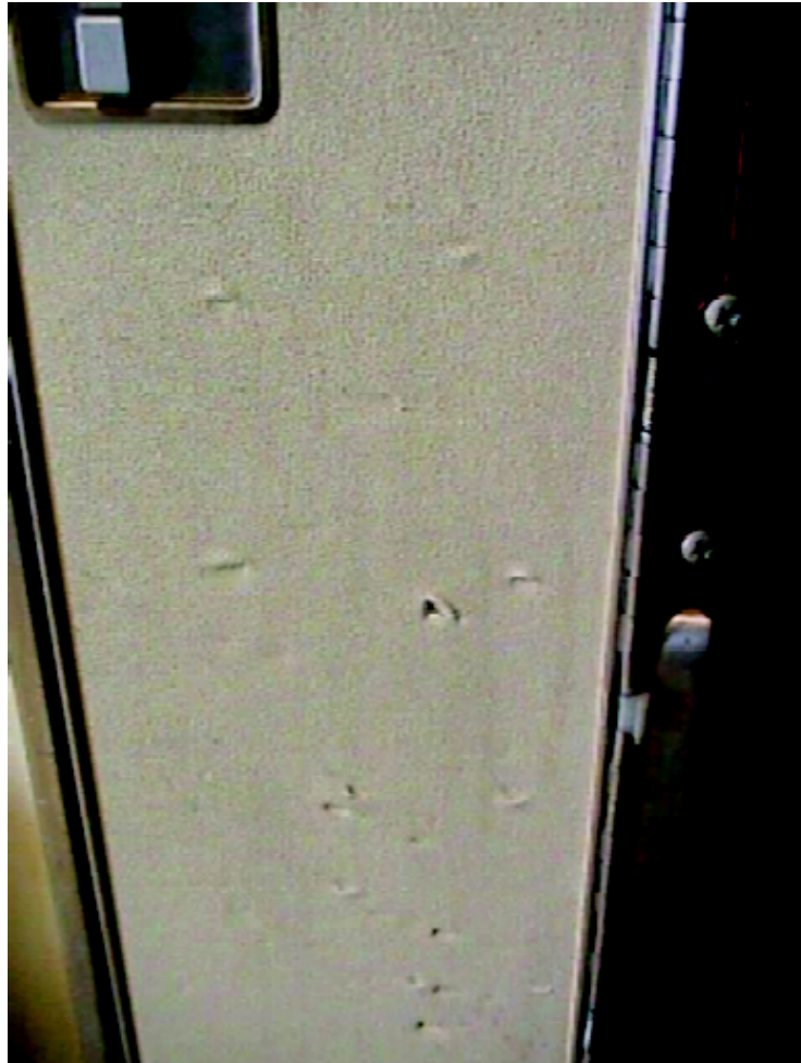
Extensive Damage on Tedlar Figure 6010
